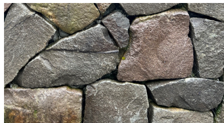
Stone Veneer @ Chimney & Foundation
