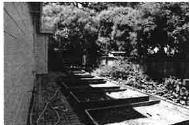
7. NORTH SIDE OF HOUSE
