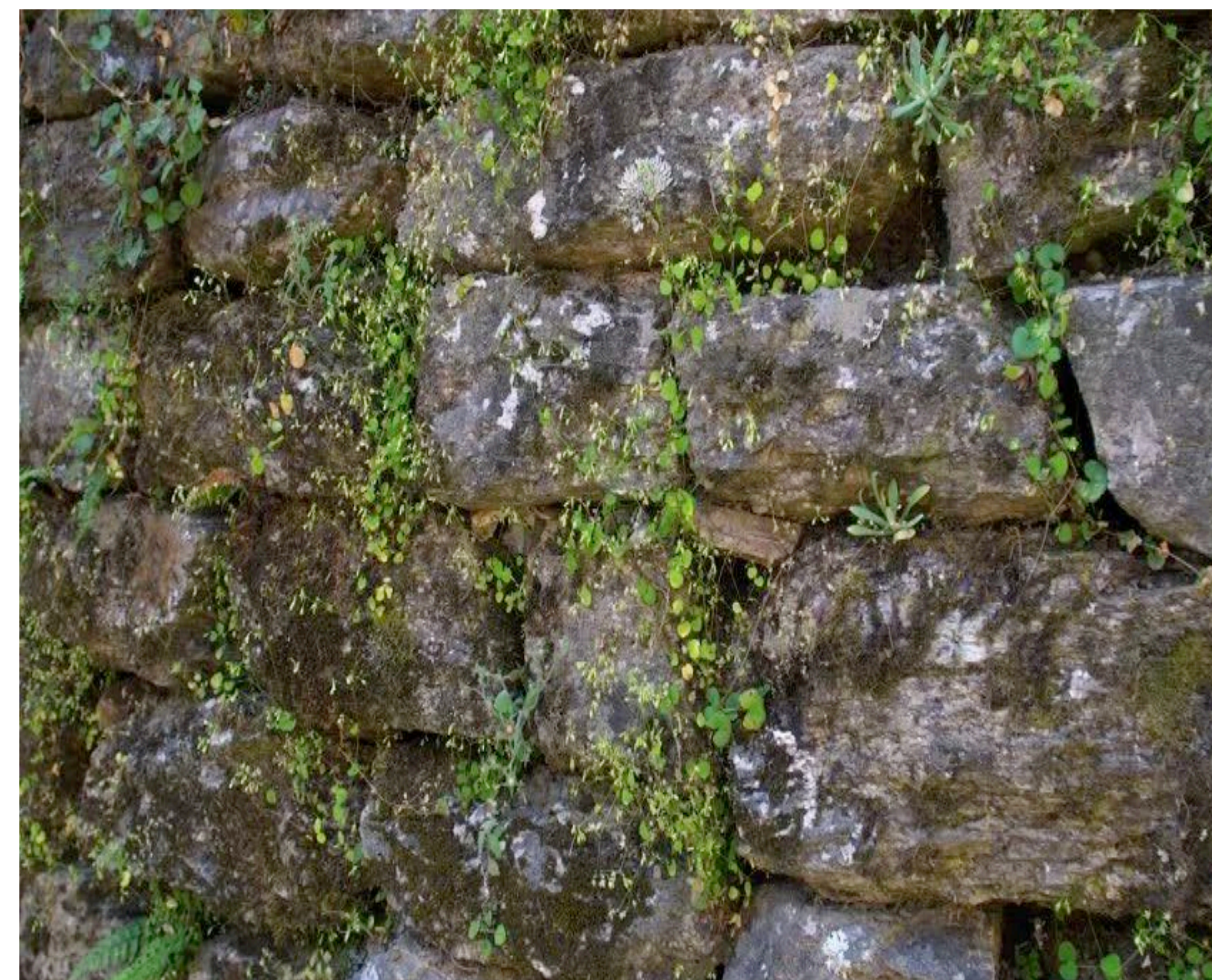
WILLOW HILL STACKED STONE WALL
