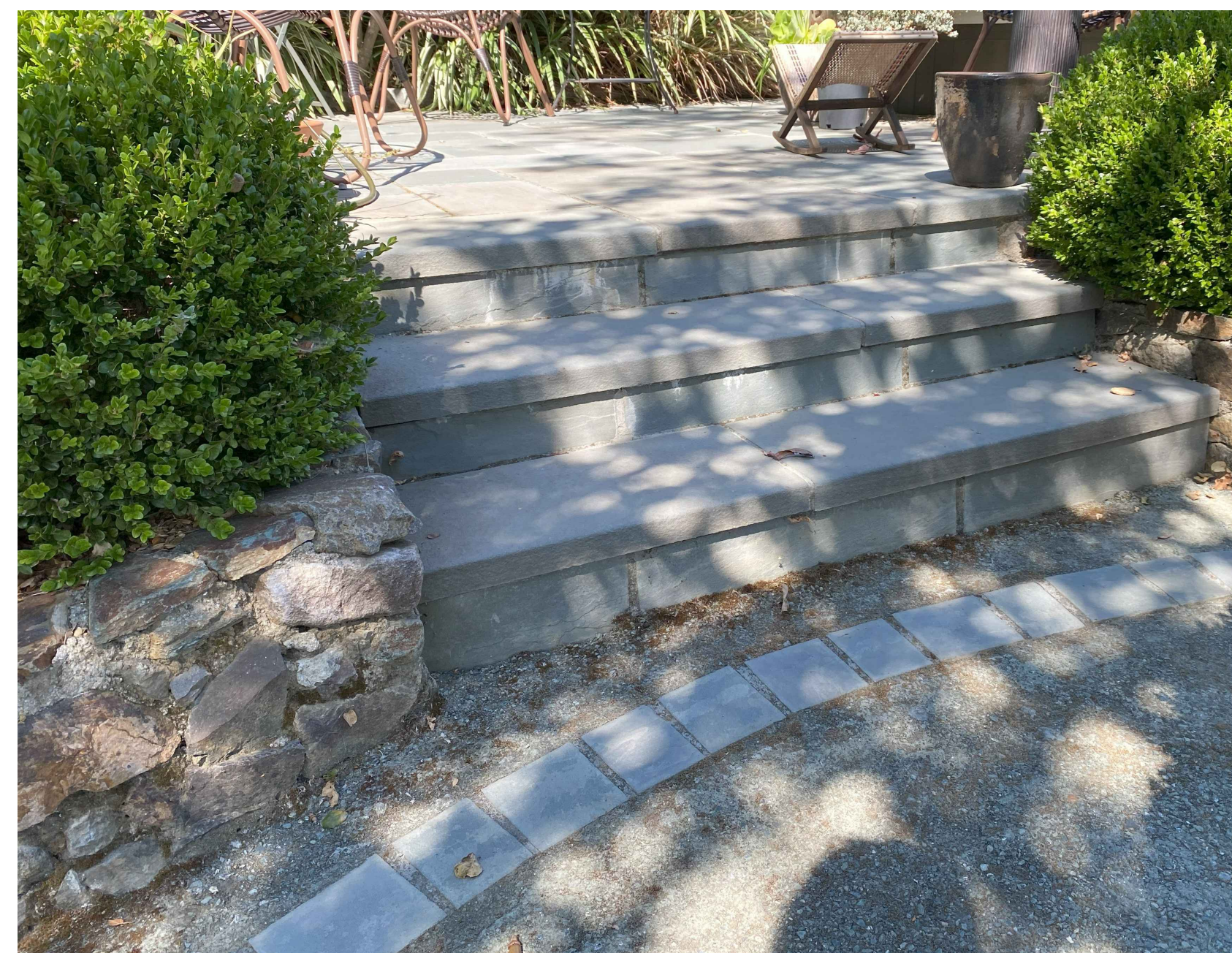
BLUESTONE PATIO AND RISERS
